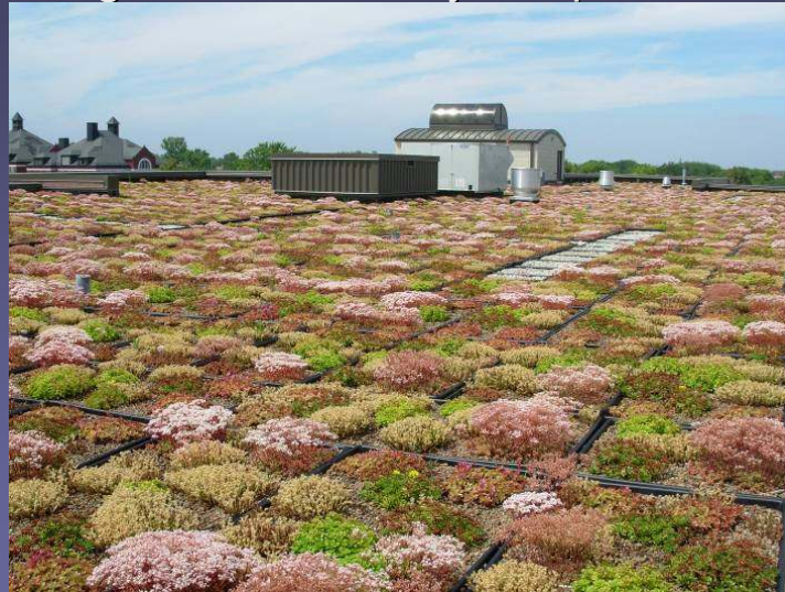
Highland Gardens, Milwaukee, WI
